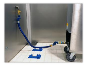
Less than ideal installation with no restraining device, high manifold inlet and low appliance inlet. A swivel has been installed on both connector ends to reduce stress and tension transferred to the connector.
